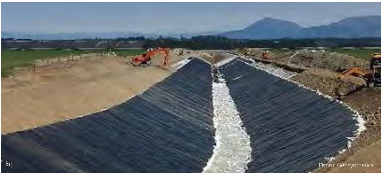
Figure 15 Canal linings a) concrete b) geotextile material
